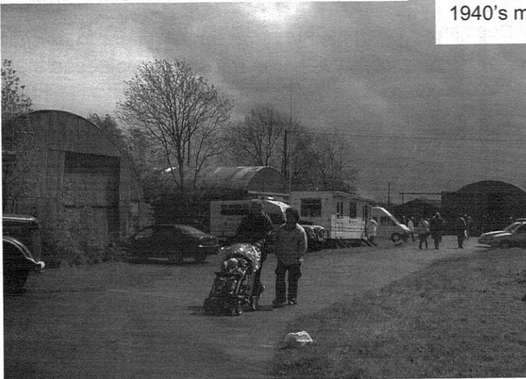
Maintenance hangar buildings still standing from WWII air operations.
